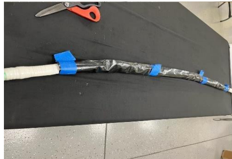
Unplug prior to pulling into pipe
