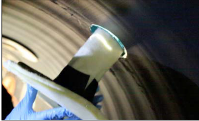
Figure 5: Lapel Liner inserted into service line
