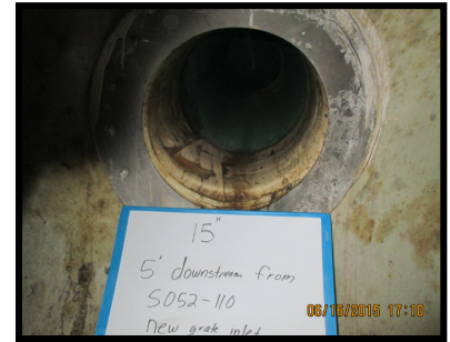
Figure 12: 15 inch cured Lapel Liner Installation
