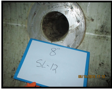
Figure 10: 8 inch cured Lapel Liner Installation
