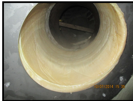
Figure 9: Cured Lapel Liner Installation
