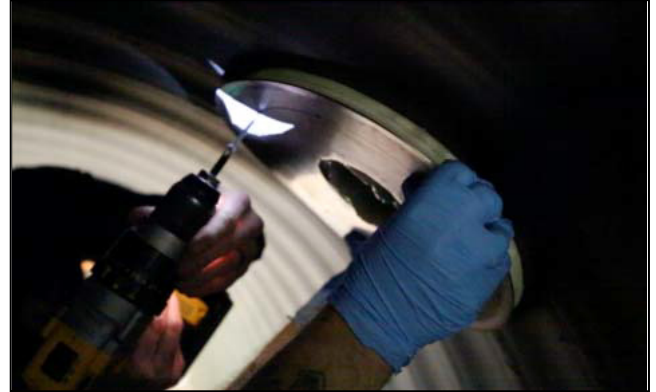
Figure 6: Anchor installation onto the brim through the steel ring
