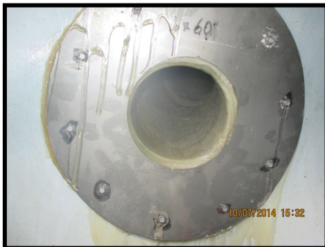
Figure 8: Cured Lapel Liner Installation
