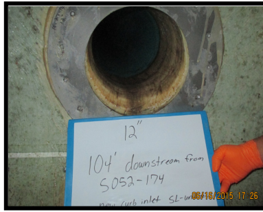
Figure 11: 12 inch cured Lapel Liner Installation
