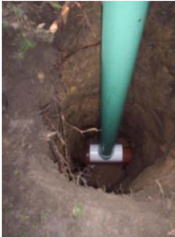
Figure 5: Hydro excavated borehole
