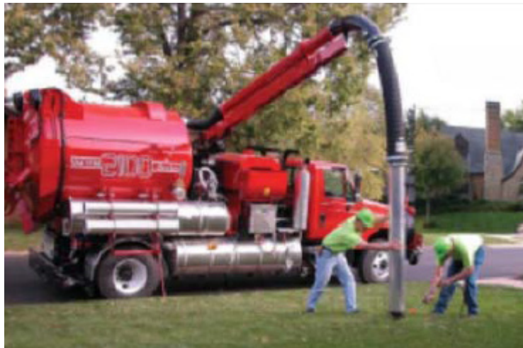
Figure 4: Vacuum excavation equipment
