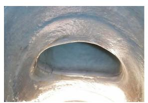
connection) and the lateral pipe so both the lateral pipe and main connection is renewed. The entire installation is made remotely from the main pipe with absolutely no digging.
