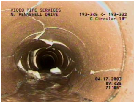
Figure 5 Structurally Compromised Pipe
