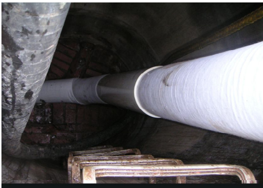
Figure 10: CIPPL Restrained Pipe Sample
