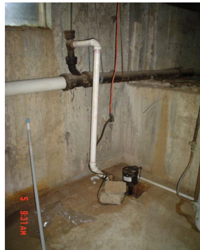
Figure 4: Illegal Sump Pump
