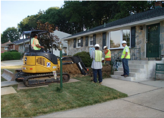
Figure 13: Cleanout Excavation
