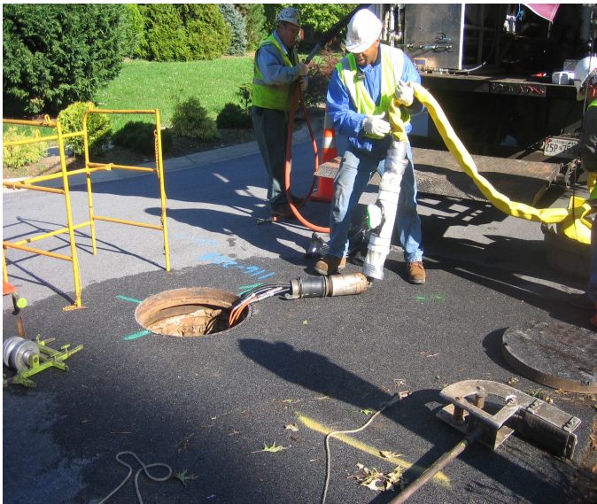
Figure 15: Inserting LCS into Mainline
