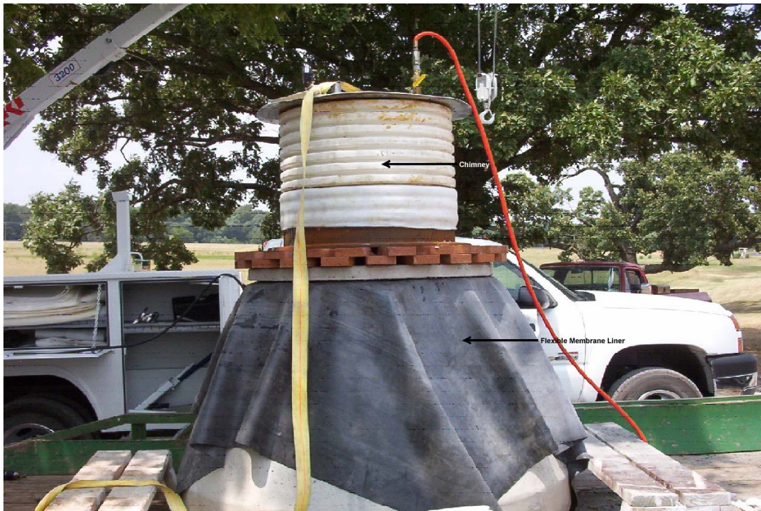
Figure 2. Installing Manhole Chimney Liner, Prior to Setting
