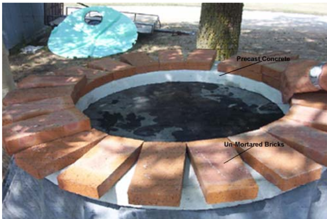
Figure 1. Constructing Manhole Chimney
