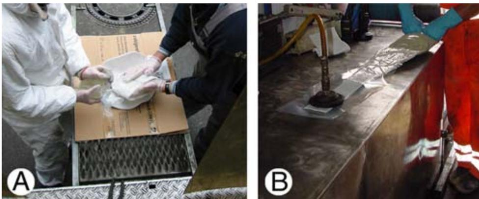
Figure 7. Top hat liner resin impregnation **A** Only manual resin impregnation. **B** Vacuum resin impregnation.
