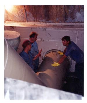
The entire installation took two days and consecutive nights. The project was cost effective and an excellent candidate for trenchless sectional repairs. The city was very pleased with the finished product of the Performance Liner®. It provided a structurally sound and corrosion resistant liner that specifically resolved the deficiencies of the siphons.
