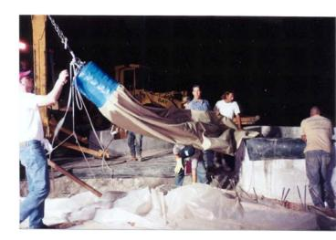
However, the resin contacts the pipe only when it is positioned at the point of repair. The linings were positioned at the beginning of the pipe at the face of the vaults wall. Air pressure was introduced into the launch tube causing the lining to invert into the damaged section of pipe. The linings were each cured within 3 hours from the time the liners were impregnated.
