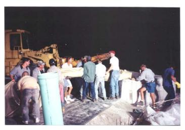
The liners required a lot of manpower to manually position the large inversion tubes. One 36-inch x 20-foot repair contained 775 pounds of resin plus the lining tube and inversion launch tube for a total weight of nearly 1,000 lbs. The liners were vacuum impregnated onsite inside of a refrigerated semi trailer. A translucent inversion bladder surrounds the lining tube.
