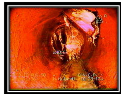
Figure 4: Protruding Hammer Tap
