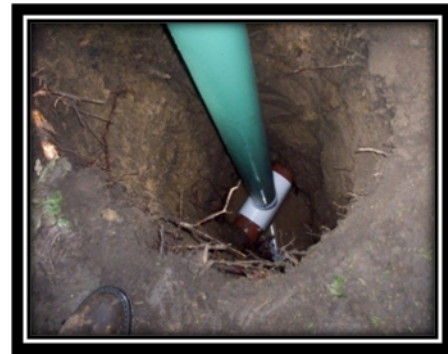
Figure 9: 20-inch DIA. Borehole
