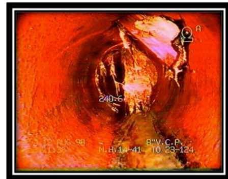
Figure 10: Protruding Hammer Tap
