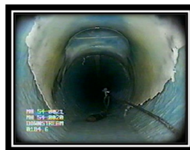
Figure 1: Delaminated
