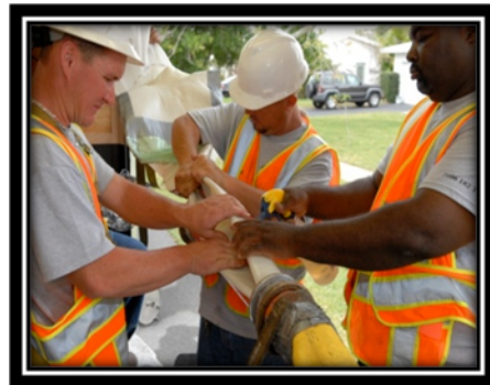
Figure 12: Inserting Liner/Bladder
