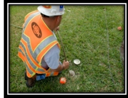
Figure 5: Clean and Inspect
