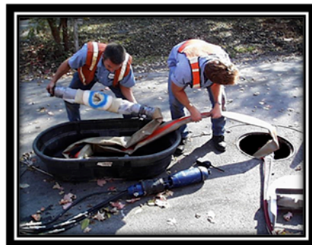
Figure 14: Inserting Launcher
