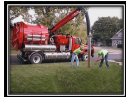
Figure 8: Vacuum Excavation
