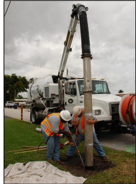
Figure 14 Shows the Minimally Disruptive Vacuum Excavation Process
