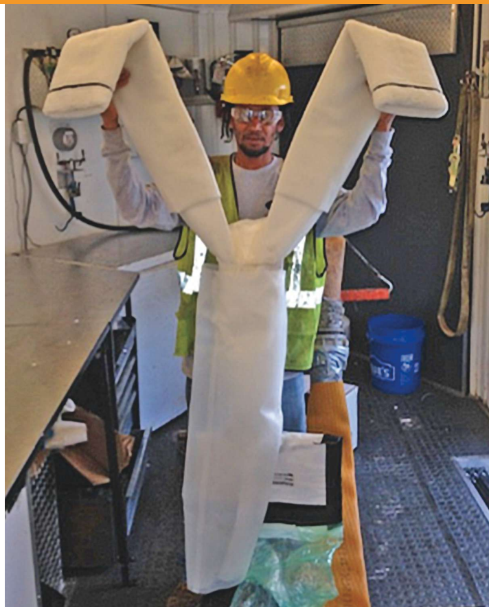
Full-Hoop Lateral Connection Liner outfitted with Compression Gasket
