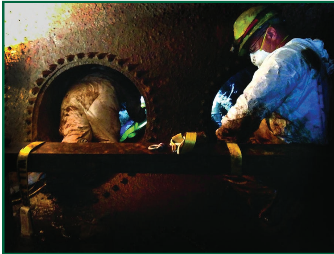
A complex pipe repair in New York's Tomhannock Reservoir
