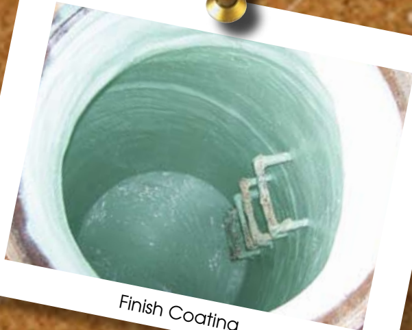
Channel, Bench, Walls & Cone
