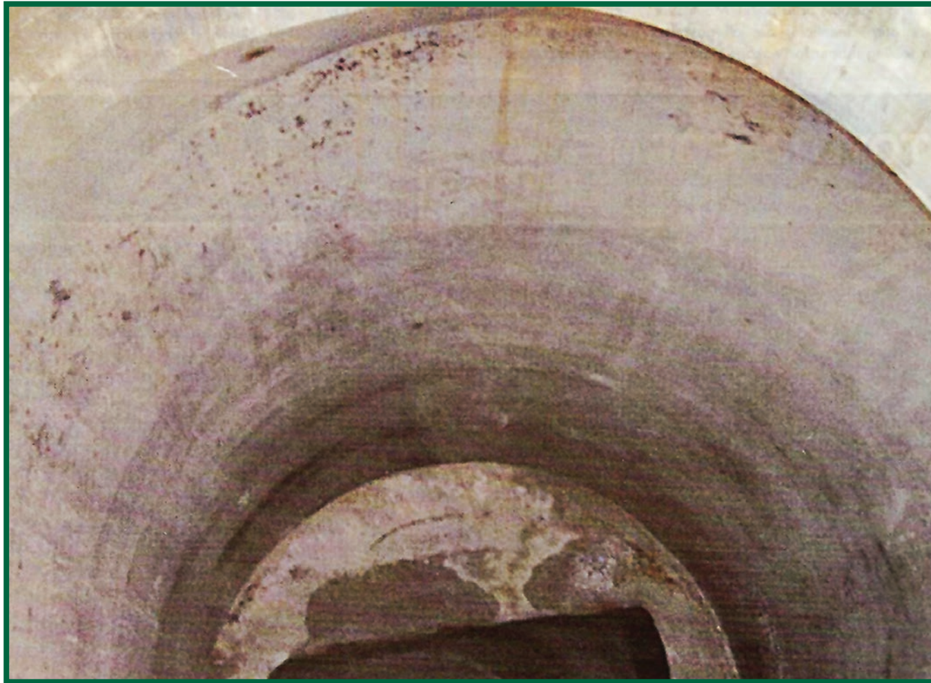
Nine-Year Test for Corrosion Protection Proves Benefit of Con mic Shield® Additive in Concrete
