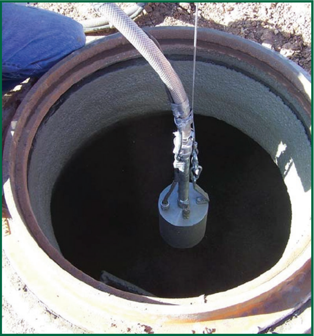
The SpinCaster makes 20 to 30 passes through the center of the manhole's axis.
