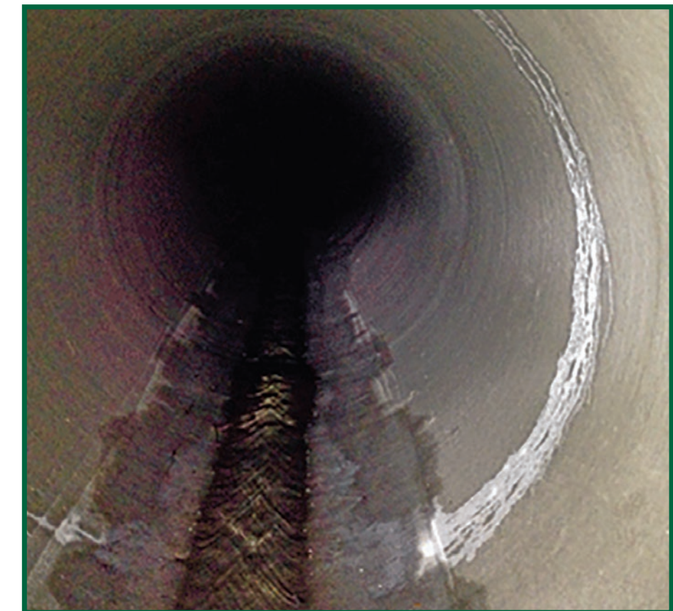
As of July 2015, AWC has completed work on four of the seven highway culverts using the centrifugally cast concrete pipe (CCCP).
