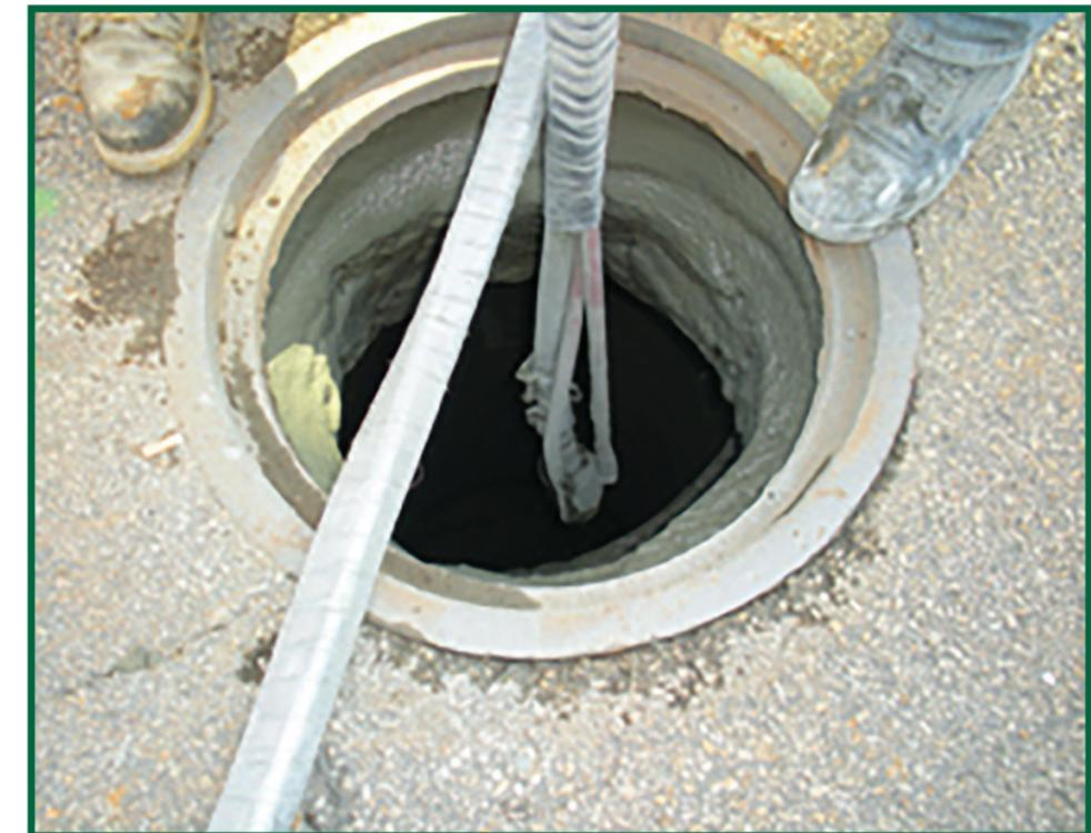
**A variety of cementitious products were evaluated and Permacast MS 10,000 made by AP/M Permaform was selected for all manhole and catch basin relining.**
