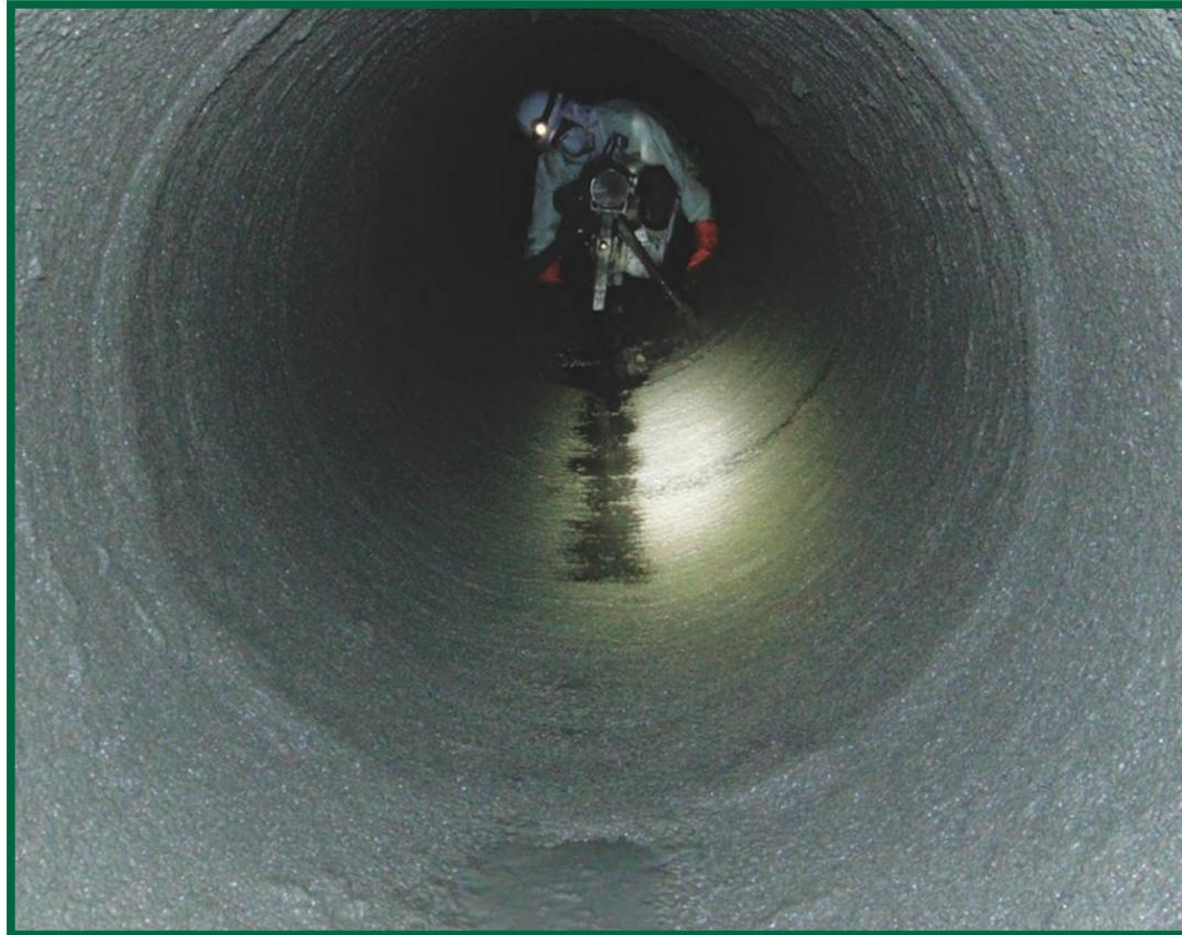
Rockland County in southern New York called for major sanitary sewer interceptor projects. The county has completed its second project, which required rehabilitating a failing sanitary sewer interceptor and pipes using cost- and labor-efficient means without disrupting rail or the New York state highway traffic overhead. In addition, the project aimed to prevent future microbiologically induced corrosion.
