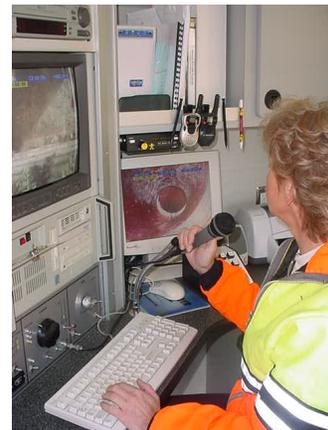
Figures 10, 11: Existing pipe being flushed and televised just before the liner installation
