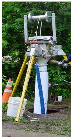
Typical installation tools for mainline installation of CIPP
