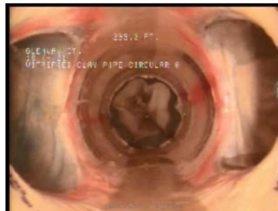
Fig 10. Continuous CIPP Siamese Lateral Connections
