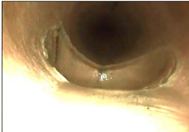
Fig 12. View from Cleanout of Bullheaded CIPP Tee at 6 o'clock
