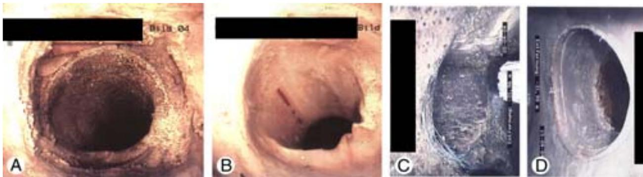
Figure 9. Repair results of construction site investigations. **A** Initial situation before repairing with a top hat liner. **B** Repair result with top hat liner. **C** Initial situation before repairing with a robotic system. **D** Repair result after repairing with a robotic system.
