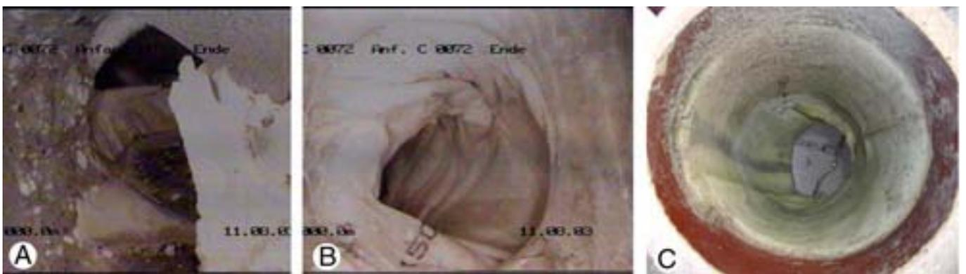
Figure 6. Examples of visually unsatisfactory repair results on extreme damages **A** Robotic system - view from the main pipe. **B** Top hat liner - view from the main pipe. **C** Top hat liner - view into the connecting pipe (after disassembly).
