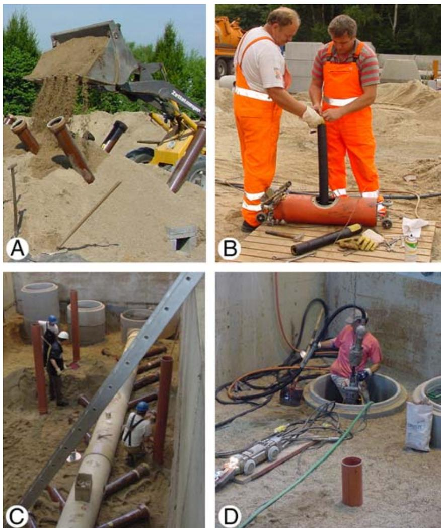
Figure 1. Test section construction and repair execution. **A** Construction of the outdoor sections. **B** Preparations for repairing the outdoor sections. **C** Test section construction on the large-scale test stand (6m x 6m x 15m). **D** Repair execution on the large-scale test stand.
