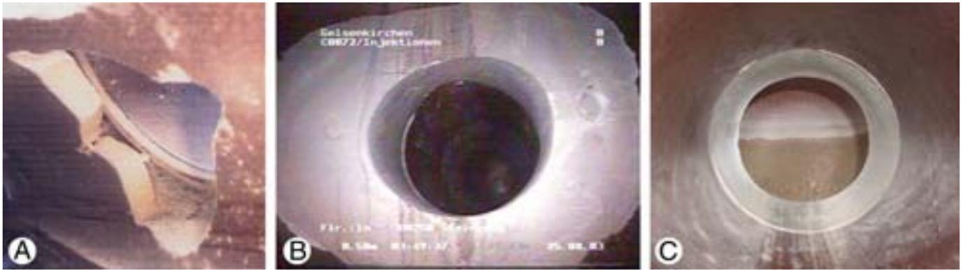
Figure 2. Standard damage for robotic systems and example of a visually satisfactory repair result. **A** Initial situation. **B** View from the main pipe. **C** View into the connecting pipe.
