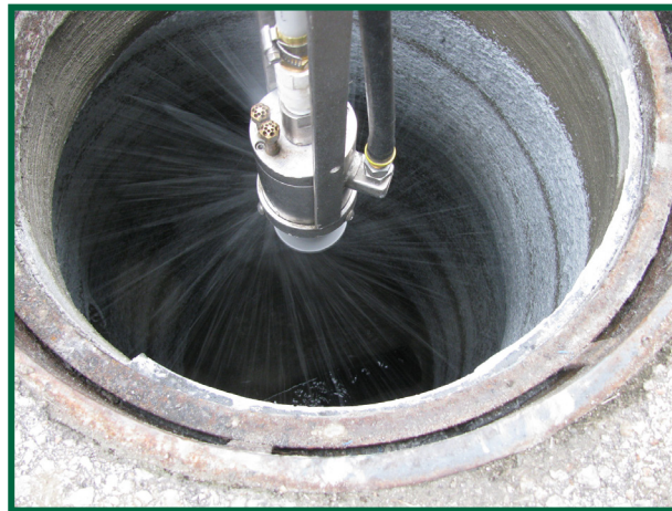
SpinCaster™ applying COR+ROC®
