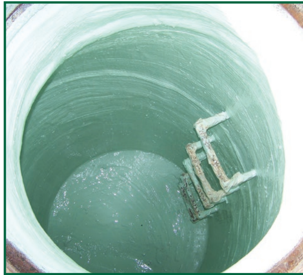
Manhole coated with COR+GARD®
